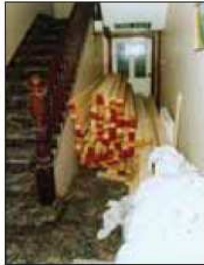
Figure 9: A blocked corridor with incorrect signage
